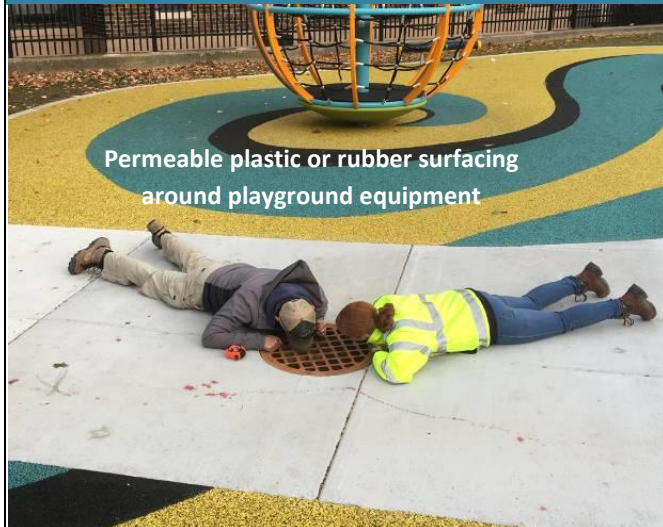
Runoff can pass through holes and gaps in the surface and drain down into and filling up the stone reservoir below.
