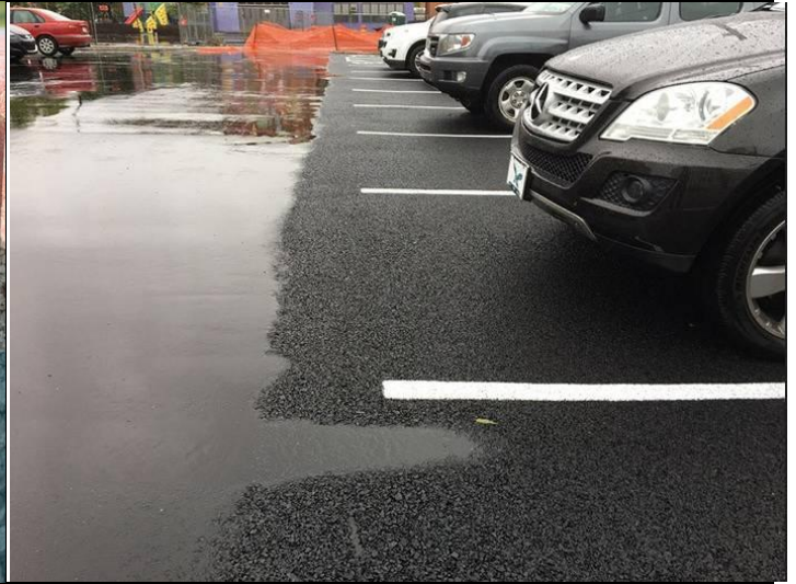
Porous asphalt used here in parking stalls (on right) and traditional asphalt used in drive aisle (on left).
